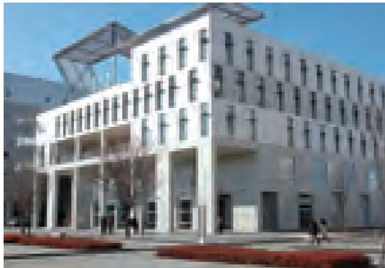
■ New IPMU building
